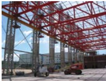
Designing a structure so that work does not need to be performed at height will prevent fall incidents e.g. lifting and erection of a hangar's roof truss.
