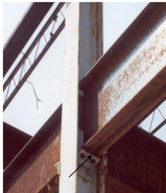
Design safety seats (see arrow) at column connections. The safety seats eliminate hanging connections making the connection process easier.
