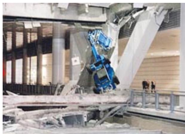
Figure 2 Structural collapse from weight of equipment
