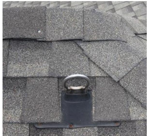
Figure 2 Residential roofing has a high incidence of falls. Installing residential roof anchors provides a place for workers to tie off.
