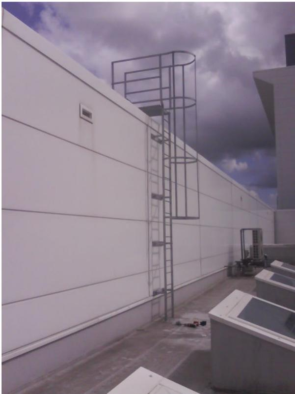
Fixed ladders should be specified to access a work platform, mezzanine, upper level, or a roof.
